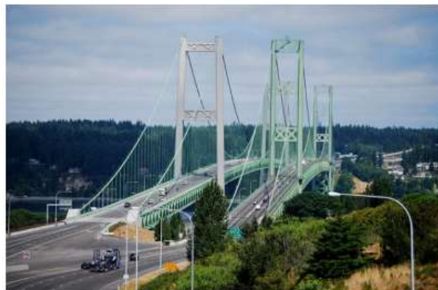
Fig. 3: Tacoma Narrows Bridge, June 14, 2008 (Source: WSDOT)
