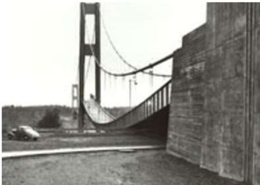
Fig. 13: M3-5: Sagging east side stretch (Source: GHM, Bashford 2795)
