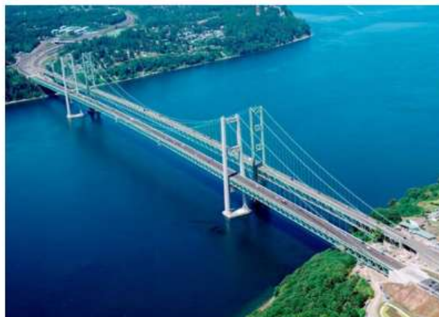
Fig. 4: Iso view of Bridge, June 14, 2008 (Source: WSDOT)
