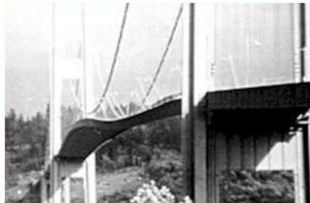
Fig. 6: Bridge Twisting (Source: GHPHSM, Bashford 2784)
