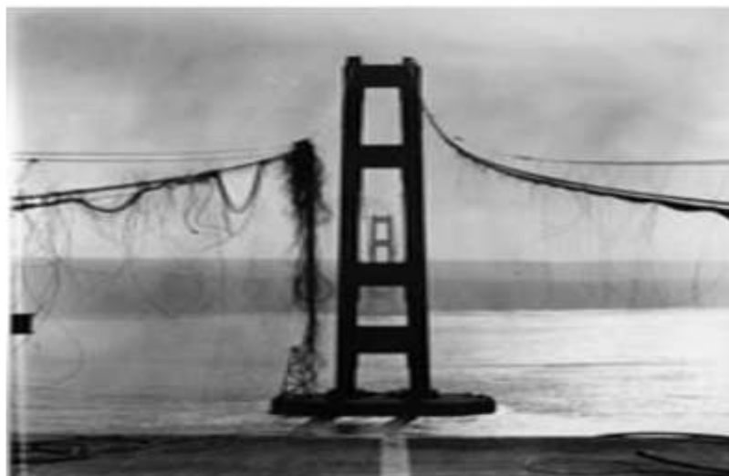
Fig. 11: View of broken wires and towers, facing west, February 1943. (Source: WSDOT)
