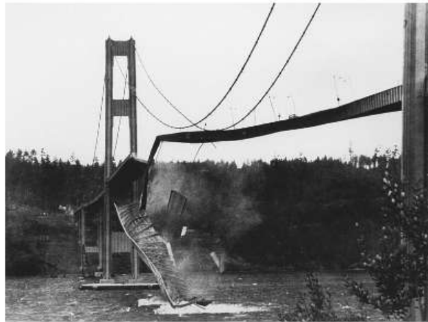
Fig. 7: On November 7, 1940, the bridge's core section collapsed into the strait below. (Source: Wikipedia)
