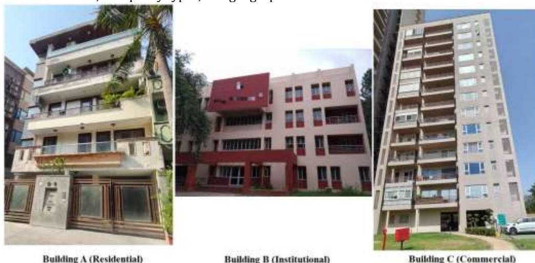
Fig. 3 Photographs of Three Case Study Buildings
